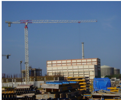
FIG 1 VIEW OF THE TOWER CRANE
