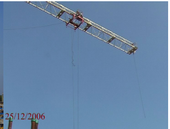
FIG 2 FAILURE LOCATION OF ROPE
